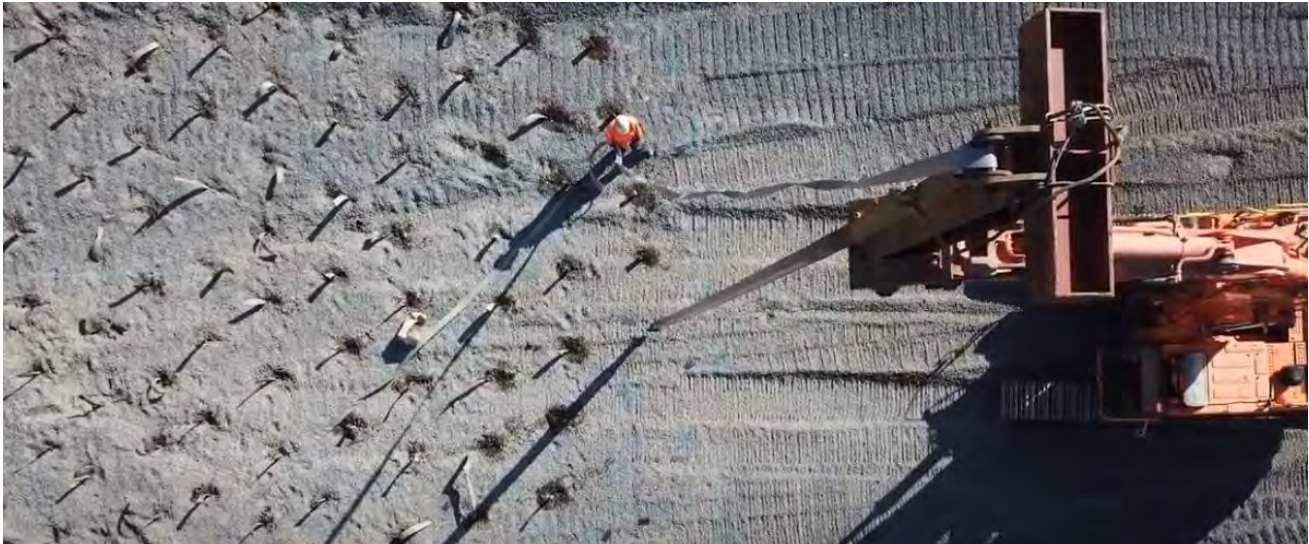
Figure 9: Photo taken from Ara Tūhono- Puhoi to Warkworth: Wick Drain Rig.
